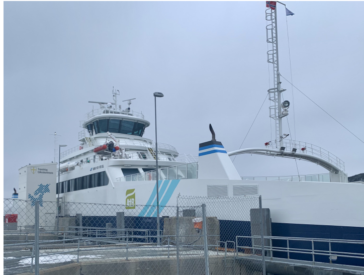
Figure 5.10: MF Lagatun charging next to one of the charge towers
