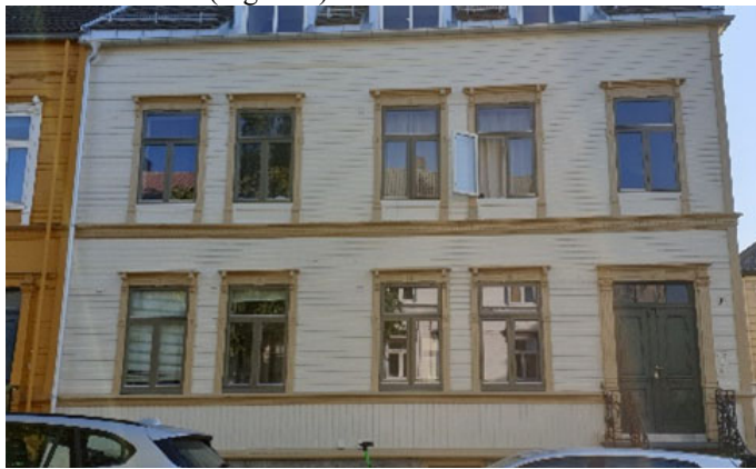
Figure 1. View of the main façade of the building.
