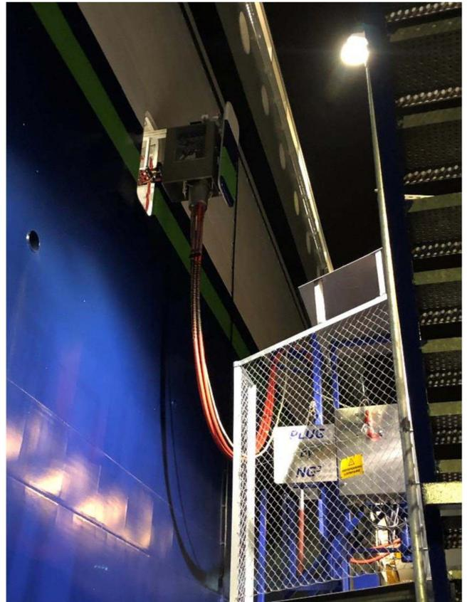
Figure 6: the typical PLUG structure and NG3 PLUG used for charging the Color Hybrid, respectively from right to left, photo: PLUG
