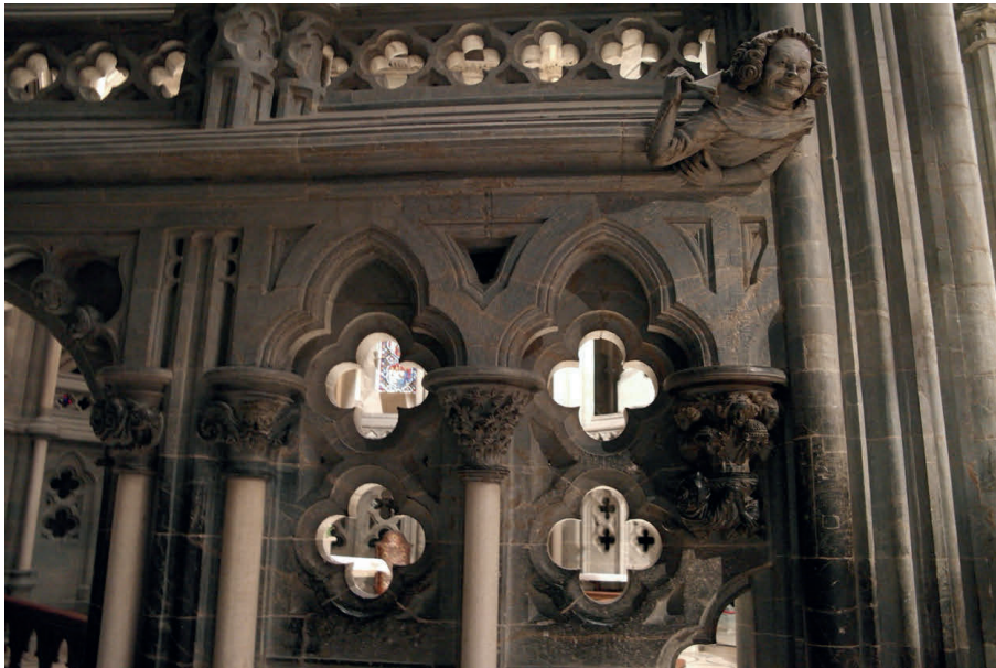
Figure 2-5: The arcade walls of the Trondheim Cathedral Octagon, view from bay 1 where the pilgrims and laypeople could enter the Octagon ambulatory. Open work tracery allows for visual access to the main altar where St. Olav's shrine was located. On the top right is a sculpture of a grinning man, removing his hood. Photo: Ingrid Lunnan Nødseth.
