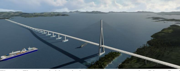
Fig. 1: Floating bridge design concept across the Bjørnafjord (COWI, 2019)
