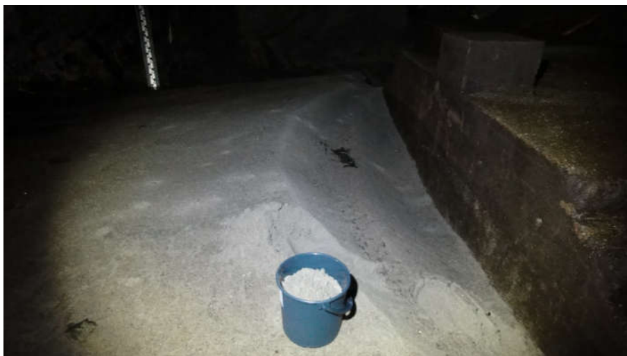
Figure 4: Deposited sand upstream the weir in the downstream end of the sandtrap
