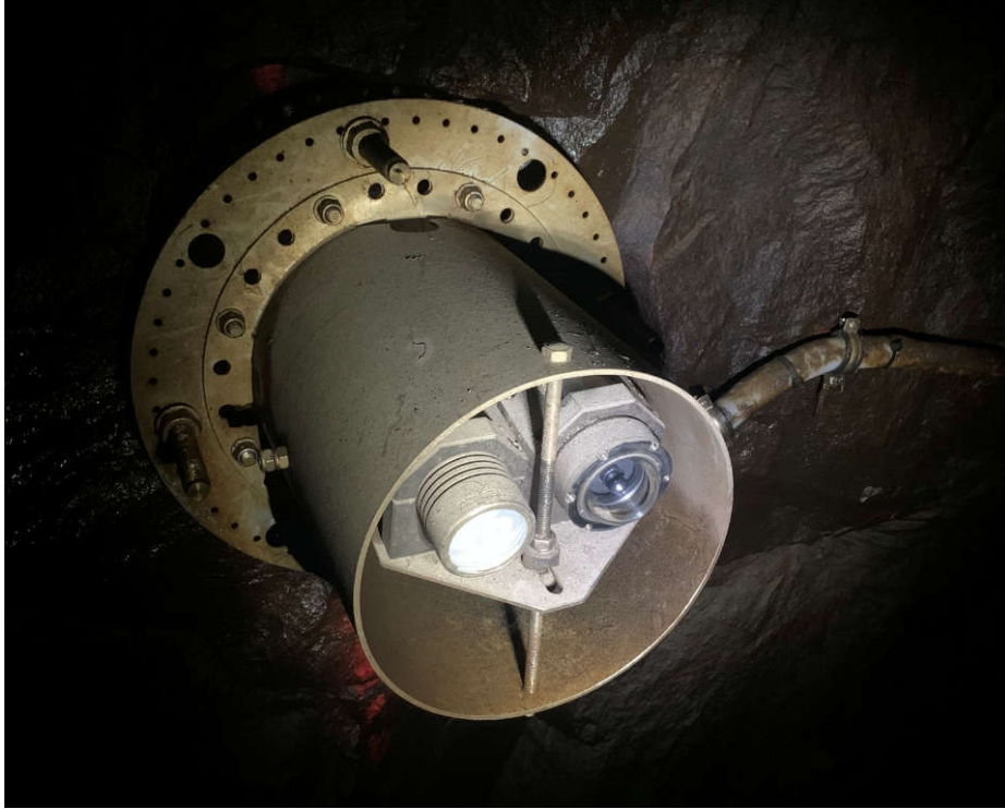
Figure 7: The sandtrap camera mounted close to the trash rack
