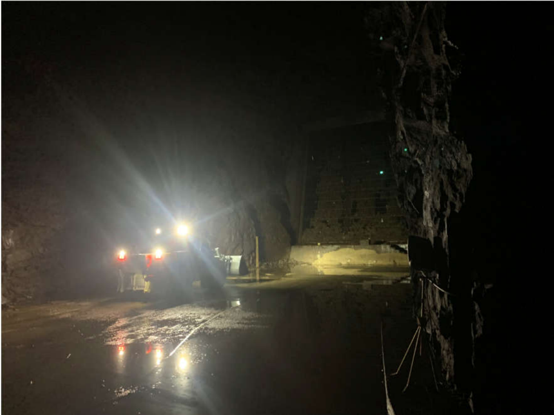
Figure 8: Cleaning of the sandtrap
