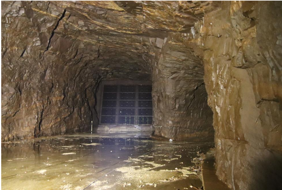
Figure 12: Flow widening at the adit (picture: Richter/TUG)
