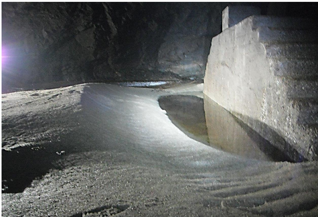
Figure 235: Sediments in the prototype at the bottom before the rake to the pressure shaft (picture: Sira Kvina)
