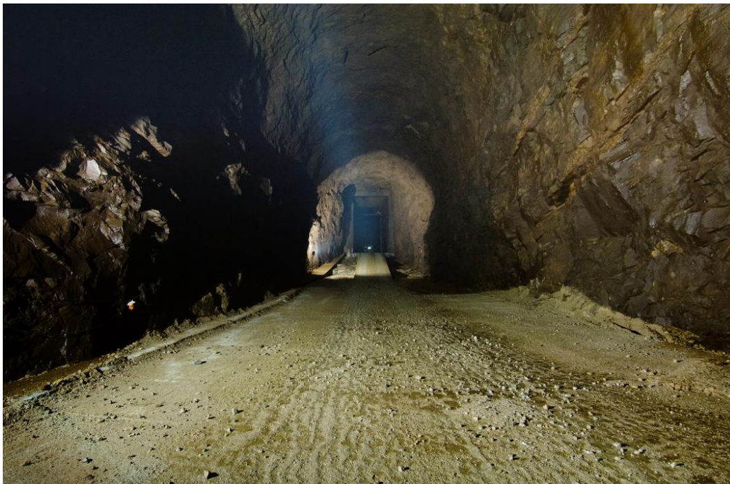
Figure 9: View inside the sand trap no3 while manual sand removing (picture: Sira Kvina)
