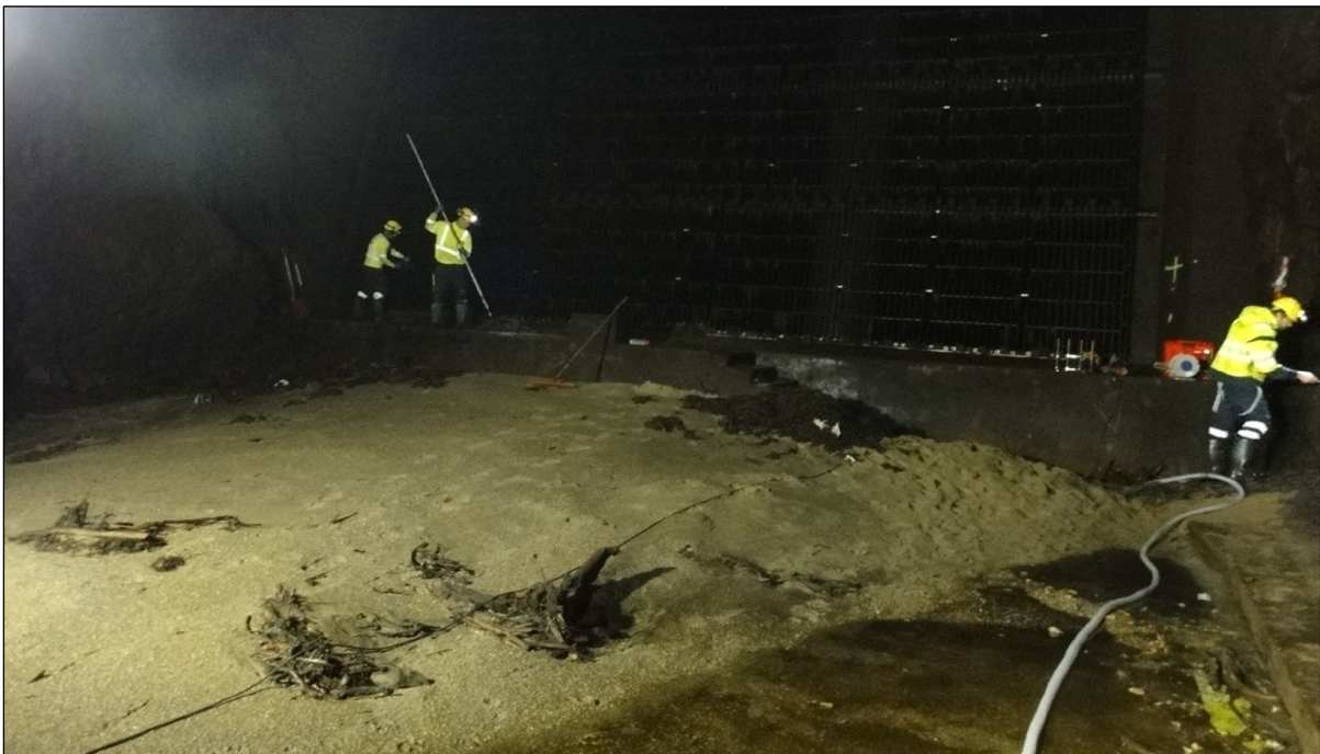
Figure 5: A view inside Tonstad sand trap III during an inspection
