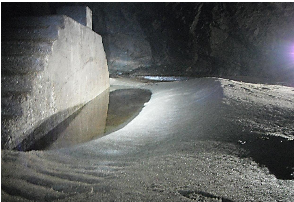
Figure 11: Sediments in front of the rake to the pressure shaft (picture: Sira Kvina)
