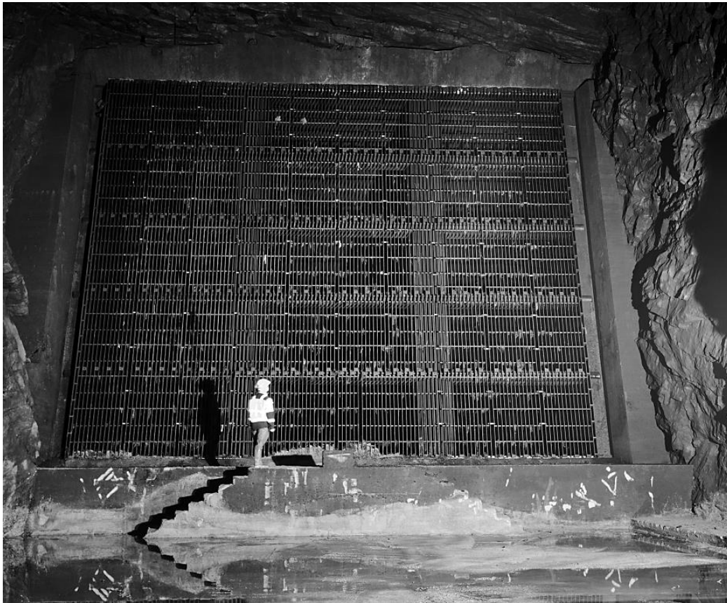
Figure 8: Rake from sand trap to pressure shaft after sediment removing (picture: Sira Kvina)
