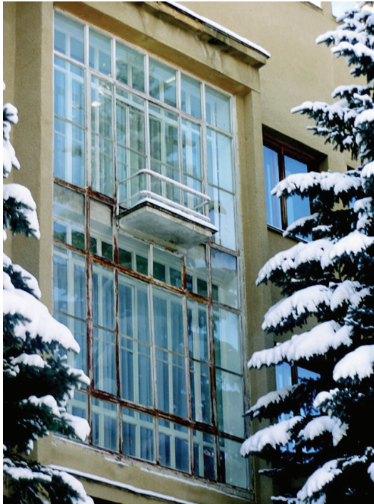
Fig. 38 Western Façade of Eastern Wing. Glass Curtain Wall and “Suspended” Balcony. (Photo Udovicki)
