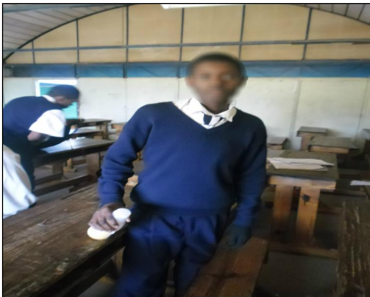
Figure 4. Showing the condition of classroom desks
