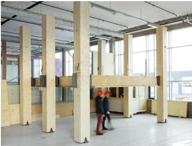
Figure 2.4. Woodsol mock-up at CVGS.
