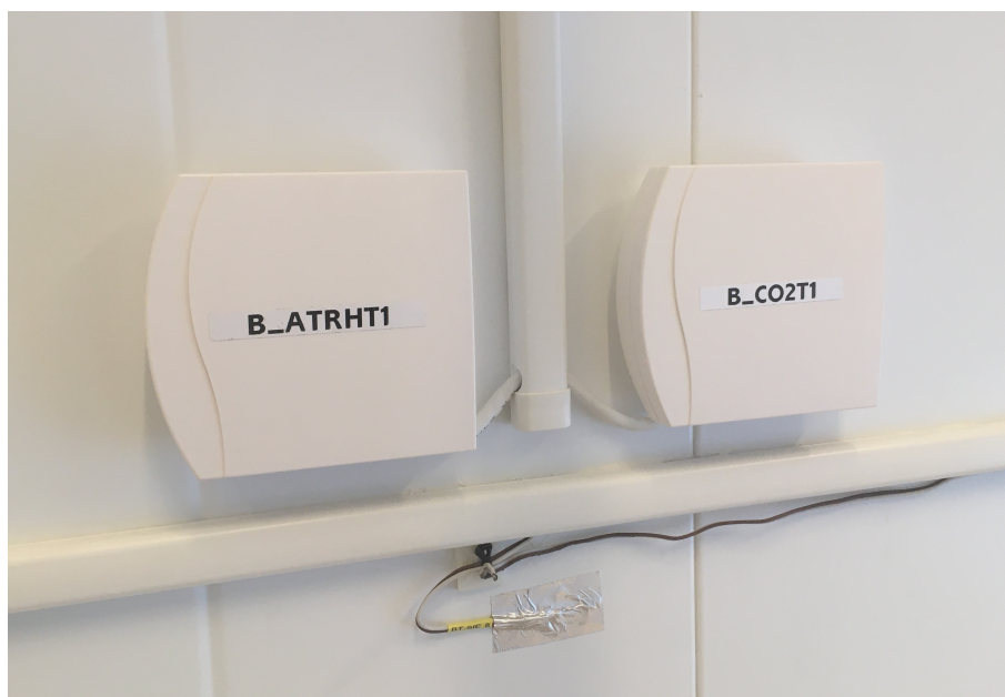
Figure 12. Sensor for temperature / humidity and CO2.
