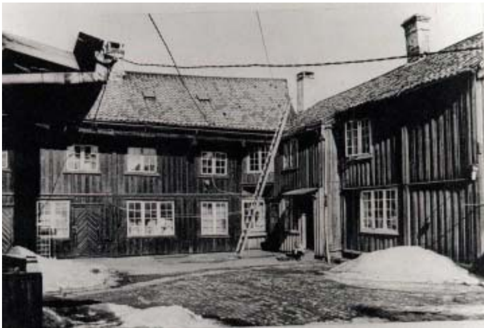
The front entrance to the dyery and the backyard of Munkegt. 24, 1967. The old building that housed the dyery was later moved to an outdoor museum in Trondheim, Byarkivet, Trondheim kommune.
