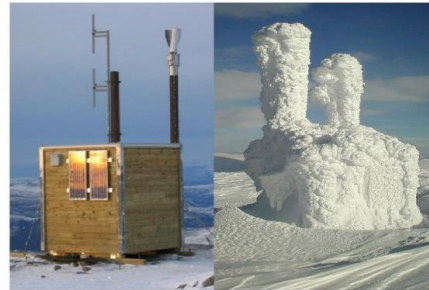
Fig. 8. Extreme ice and snow accumulation on a communications station, before (left) and after (right) accumulation. Courtesy of GETEK Energy AS (Norway).
