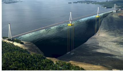
(a) TLP type floating bridge (Statens Vegvesen (2019))
