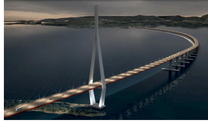
(b) Multi-pontoon floating bridge (Statens Vegvesen (2019))
