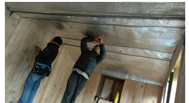
Taped joints, Beehive Lodge, Paiya
