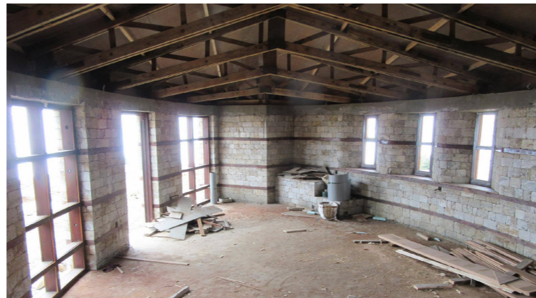
One of the buildings in Sagarmatha Next project
