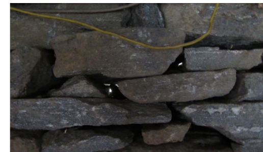
Daylight visible through dry stone wall, Beehive Lodge, Paiya
