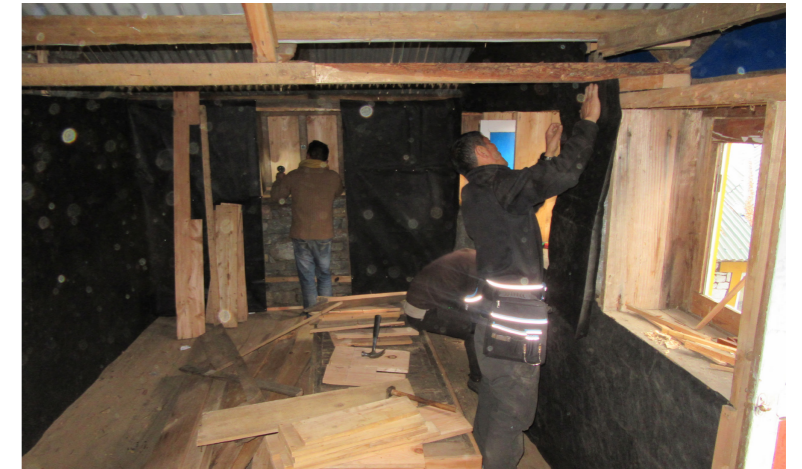
Removed timber linings to install a breathable membrane, Beehive Lodge, Paiya
