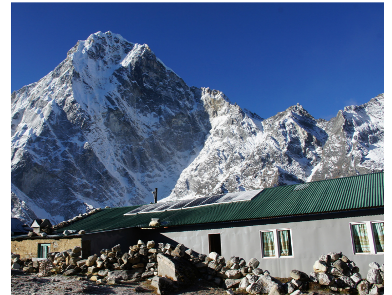
Dzongla Inn 4830m, clear skies and cold temperatures are ideal for PV panels
