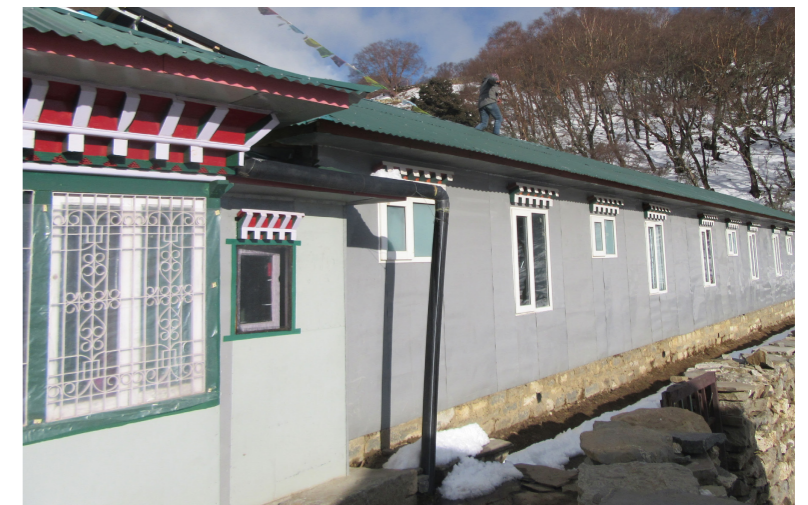
Example of flat sheet steel at Phortse Guesthouse
