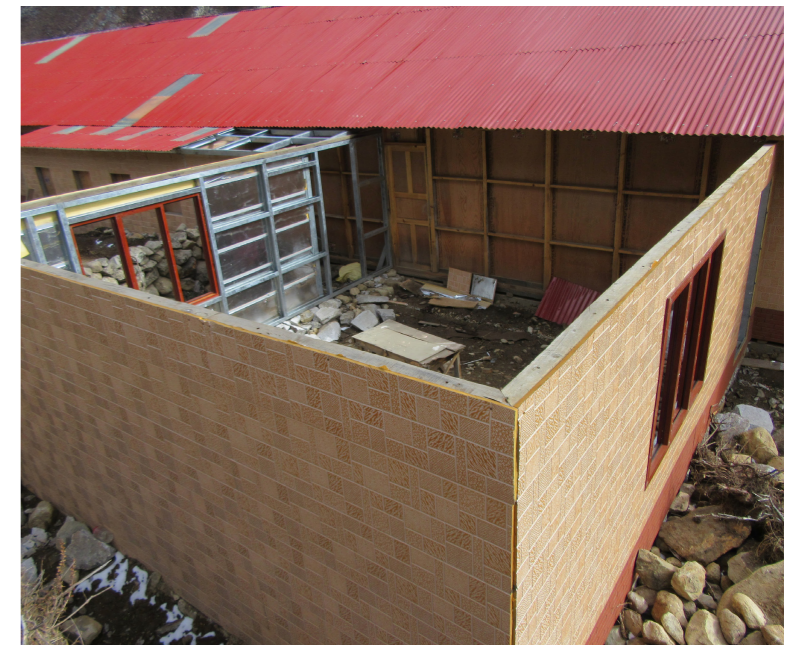
Variation of panel system with "timber head binder"
