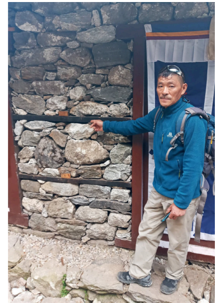
Ganga showing the horizontal timber battens built into the dry stone wall
