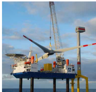
(b) HOCHTIEFS's Thor jack-up platform. Photo: hochtief-construction.com
