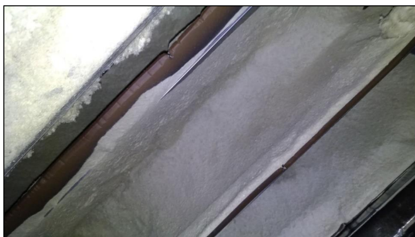
Figur 4.15: Groing i transportlukene
