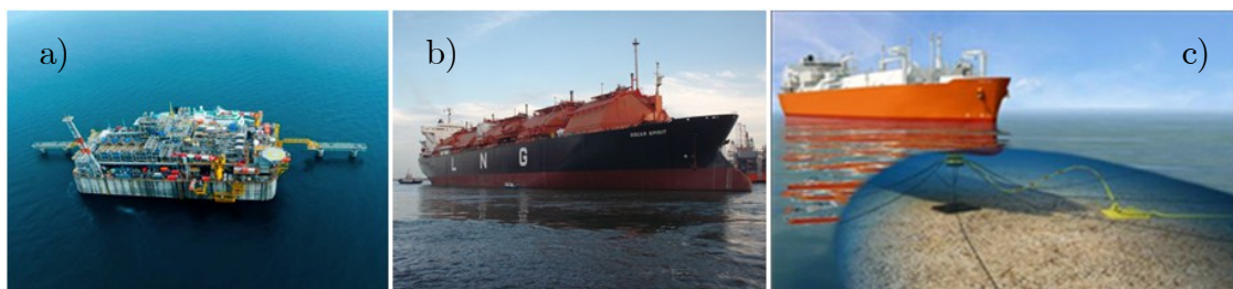
Figure 3-10: Three examples of offshore regasification units: a) Adriatic LNG terminal is the world's first gravity based LNG receiving structure. It is located off the coast of Italy, started operation in 2009, measures 47 by 88 meters and has a capacity of 8 bcm per year (about 10% of Italy's gas consumption). b) Golar Spirit is the first FSRU converted from an LNG carrier. It is located off the coast of Brazil, started regasification in 2009 and has a throughput capacity of 2.5 bcm per year. c) Illustration of Port Dolphin SRV. This vessel has a buoy connection under water.
