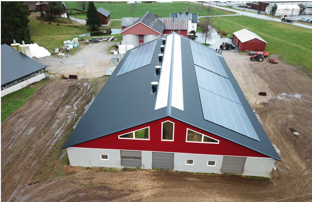
Figure 2.3: Solar energy system in Marnardal. The system is installed with 98 kWp. [27]
