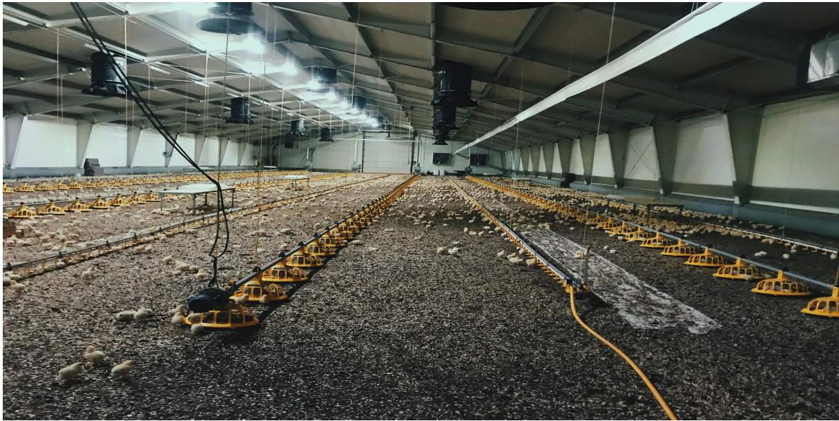
Figure 3.4: Internal view of the barn. [3]
