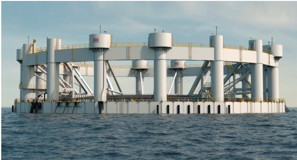
Figure 6.6: The facility AOF is a semi-submersible construction with rigid steel structure. The height of the facility is 21 m with an outer diameter of 79 m. Number of fish per cage are 600 000.[160]
