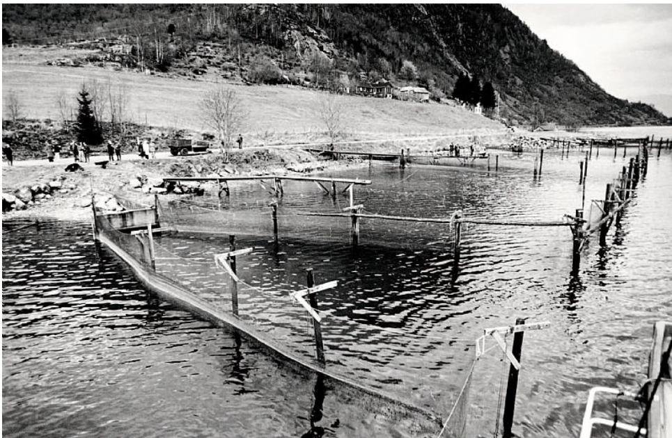
Figure 2.1: Fish caging made by linen, rigged up by wooden poles in the sea, one of the earliest technologies used for fish farming. The picture is from the 1950s and taken in Bjordal in Høyanger municipality.[14]
