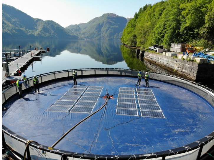
Figure 5.4: A test project for a floating solar plant, located at Osterøy near Bergen, and is supposed to supply a fish farm with electricity.[110]
