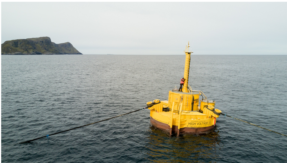
Figure 5.7: Wave-EL placed outside Runde in Sunnmøre was the first wave power technology ever to be resynchronized with the Norwegian electricity grid. The system was fully functional delivering 100 kW.[129]
