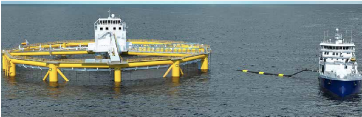
Figure 6.1: The facility Ocean Farm 1 is an independent unit with rigid steel structure. The total height of the facility is 68 m with a diameter of 110 m. The volume is 250 000 m^3 . [153]
