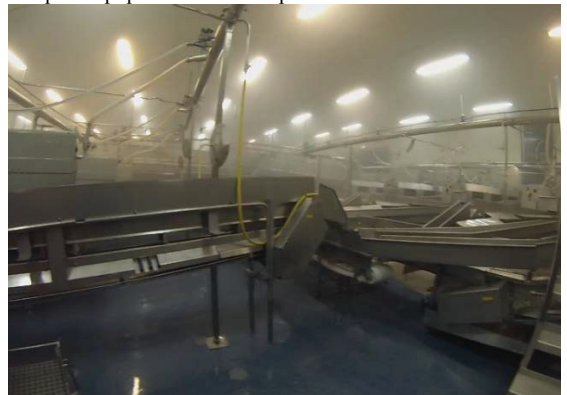
Fig. 2 Operational environment of robotic cleaning system
