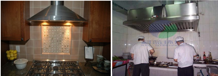
Figure 1: Kitchen exhaust hood (canopy/range hood) in a domestic kitchen (to the left) and in a commercial kitchen (to the right)
