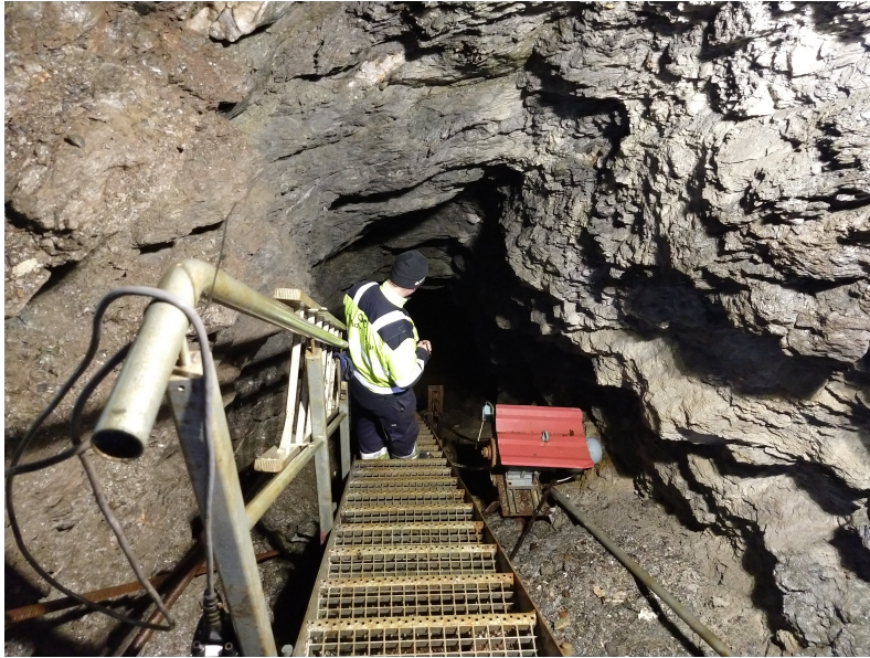
Figure 2.4: A picture from the site visit of the surge chamber at the end of the water tunnel at Simsfossen.
