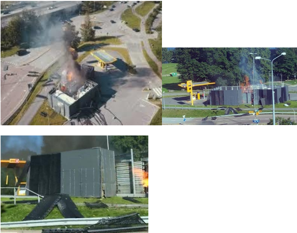
Figure 23: Photos from Kjørbo station (“Immagine incidente,” n.d.) (“accident images,” n.d.)
