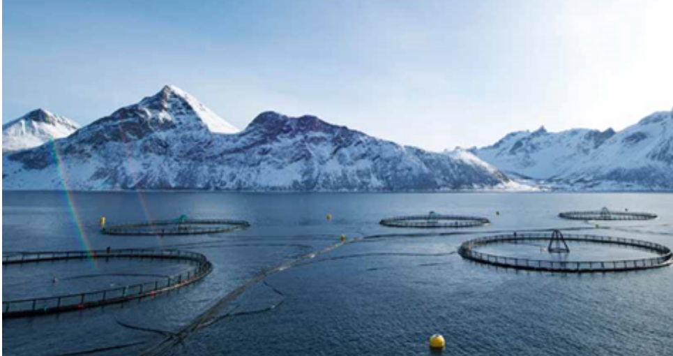
Figure 3.4.2: A circular HDPE floating fish farm. Source: The Norwegian Seafood Federation (2011)
