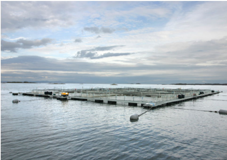
Figure 3.4.3: An example of a steel hinged fish farm. Source: AKVA Group
