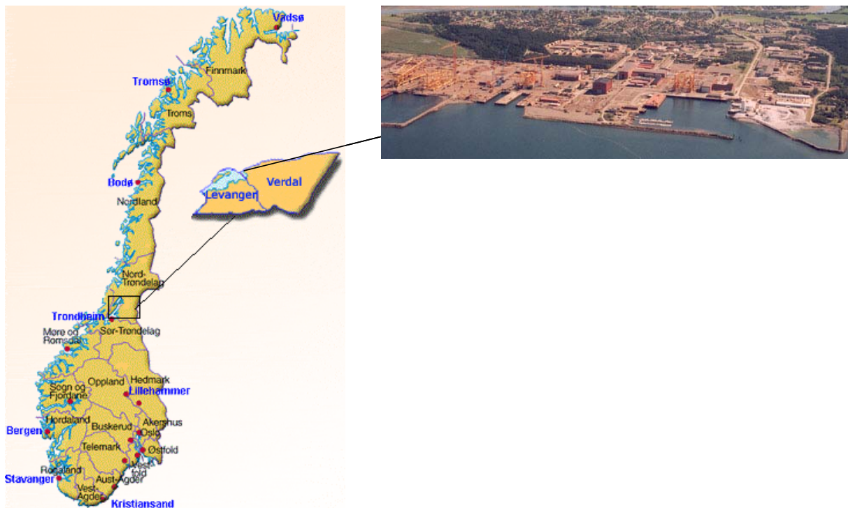
Figure 5-1: Verdal Industrial Park – view from the west
