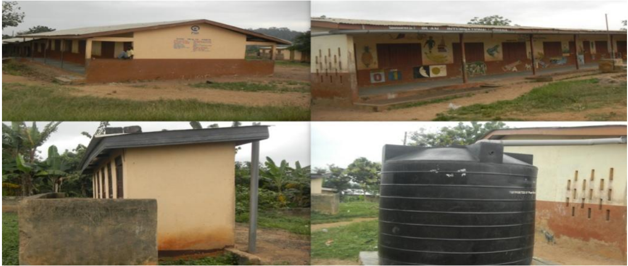
Figure 2: Plan Ghana's educational projects in the Awutu-Senya District (Source: Photos taken from field trip, July, 2012).
