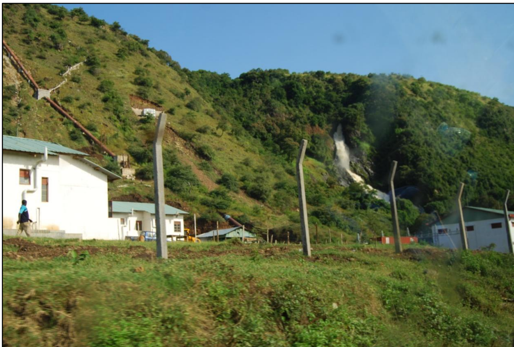
Picture 5.3: Power-plant (Private photo).
