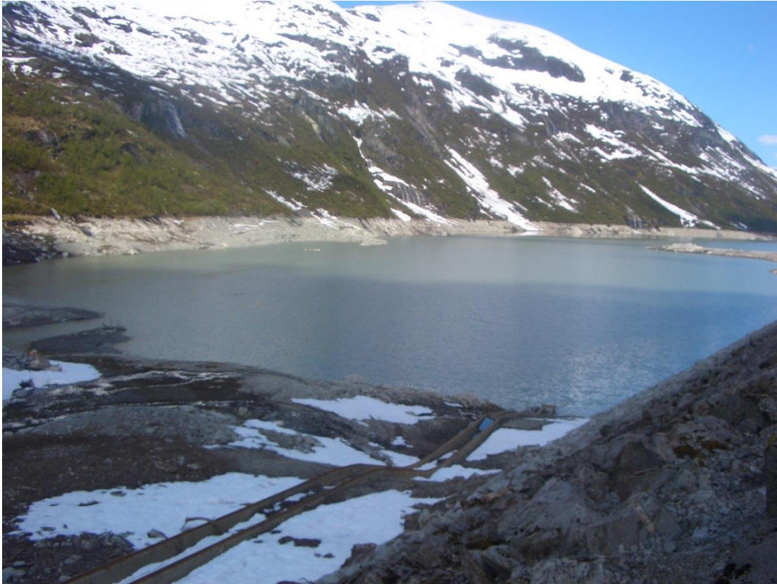
Figure 3.4: Water level in Tunsebergdammen, reservoir to Leirdøla large-scale hydropower plant. Source: Tor Haakon Bakken.
