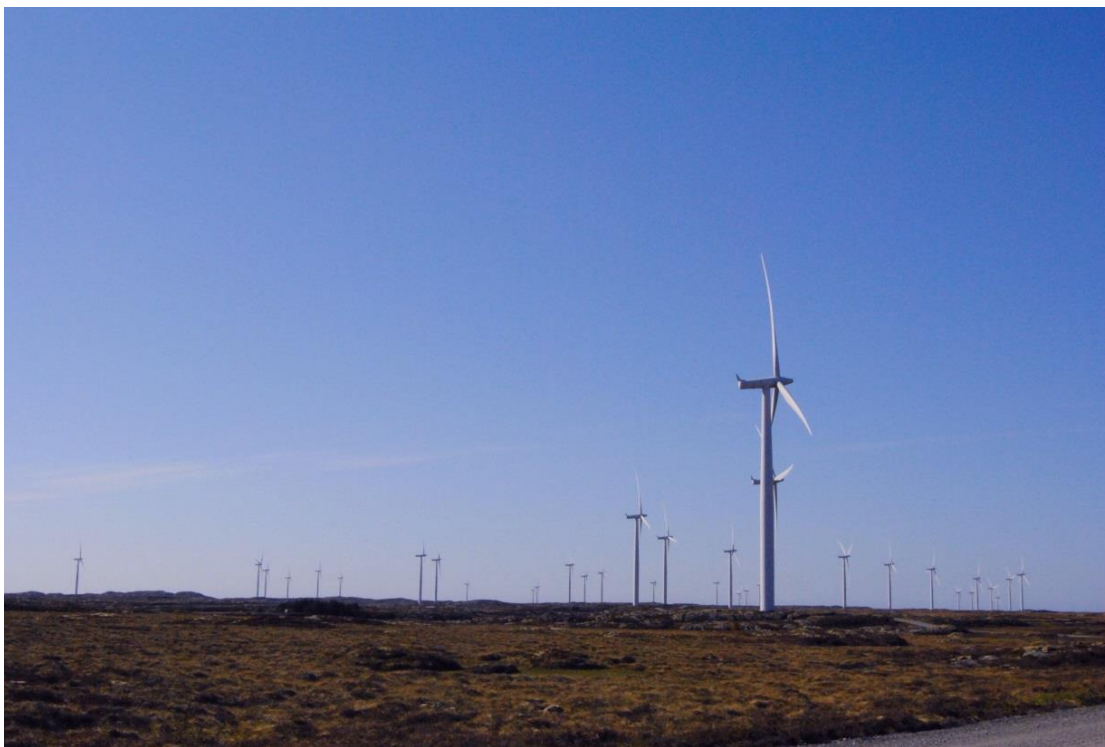
Figure 2.5: Smøla wind power plant. Source: author.
