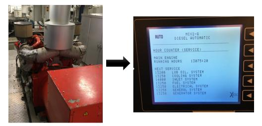
Figure 1.1: One out of three marine diesel engines on board  $\rm R/V$  Gunnerus and its predetermined maintenance intervals.
