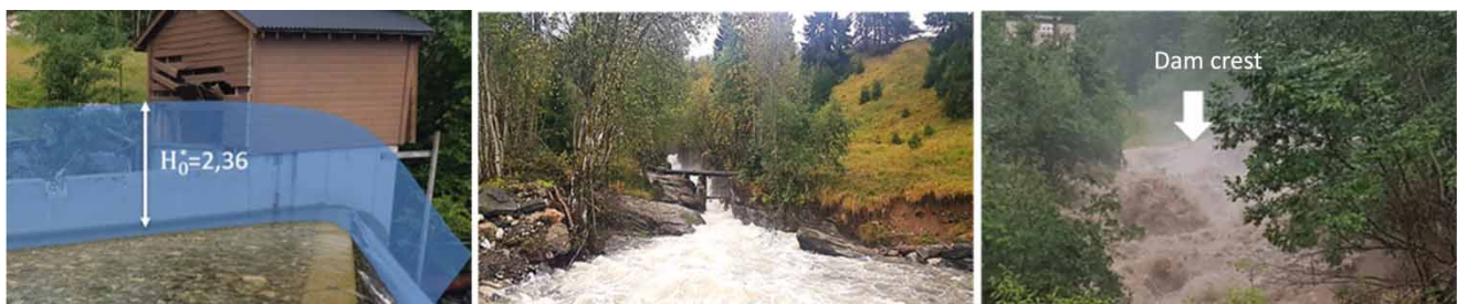
Figure 6 | Illustrated water over the crest level, and picture of upstream of the crest and of the flow over the crest during the event.
