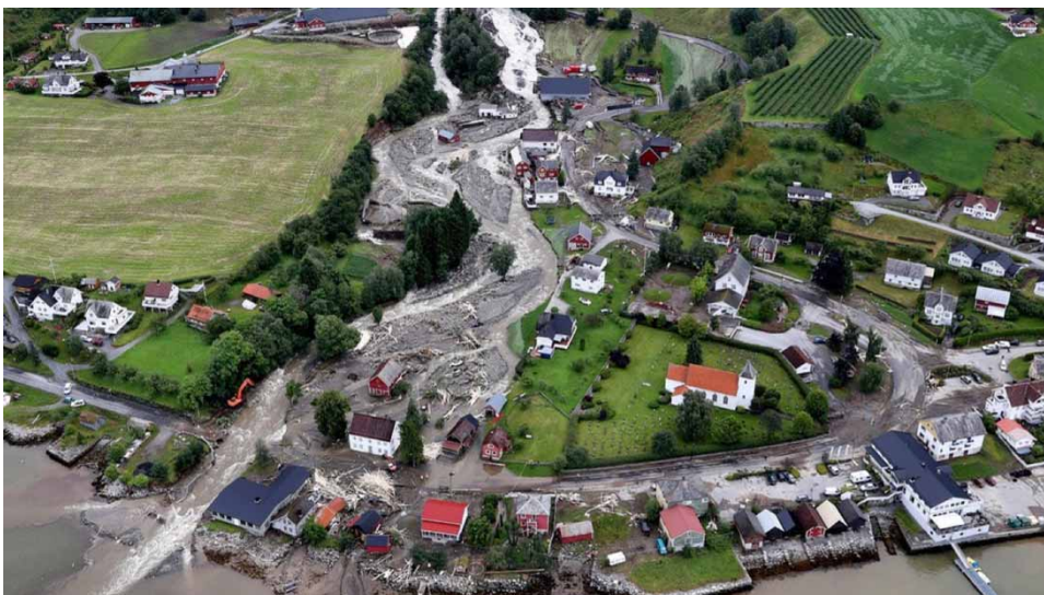
Figure 4 | Overview picture showing the new watercourse and damage caused by the flood in Utvik (source: Hallgeir Vågenes, VG 2017).
