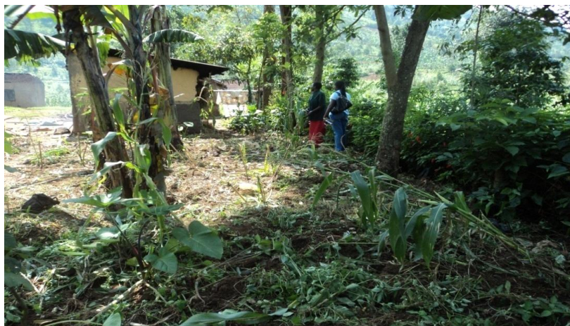
Figure 5.2: Poorly built house near a wetland.
