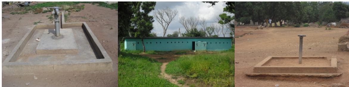
Figure 8: From left, a bore hole at Gyama New Settlement, the 24 seats toilet at Gyama New Settlement and the third is a bore hole provided at Dasaase under the Akosombo resettlement
