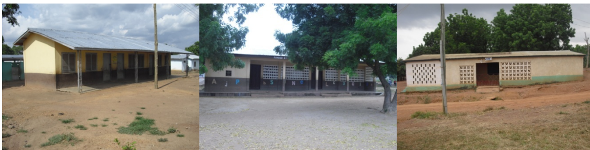
Figure 9: From left, nursery school at the Gyama New settlement, VRA resettlement trust fund primary school complex and a clinic provided at Dasaase (Senchi) resettlement under the Akosombo project.
