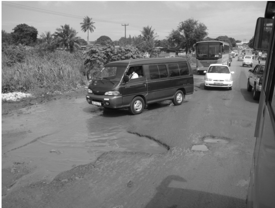
Plate 6.4 Road Infrastructure on the Kimbu-Adenta Highway. Source: Field Survey, 2008.
