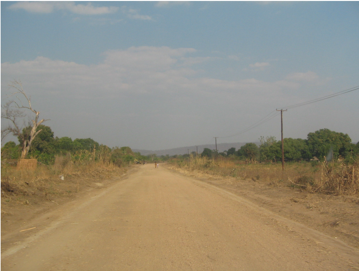
Figure 9: Mfuwe Road showing a section recently upgraded.
