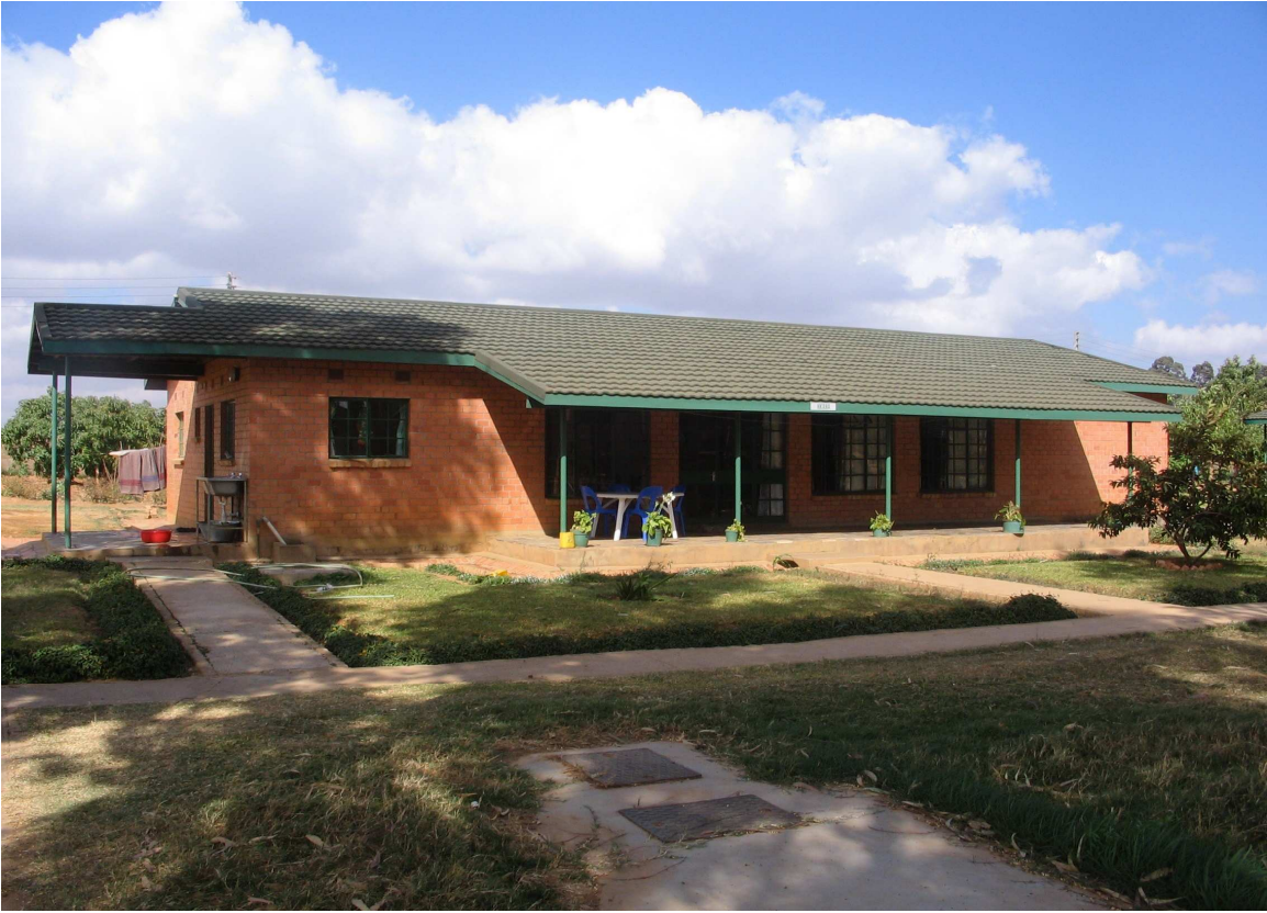
A residential house (decent shelter) for OVCs at Lusaka SOS
