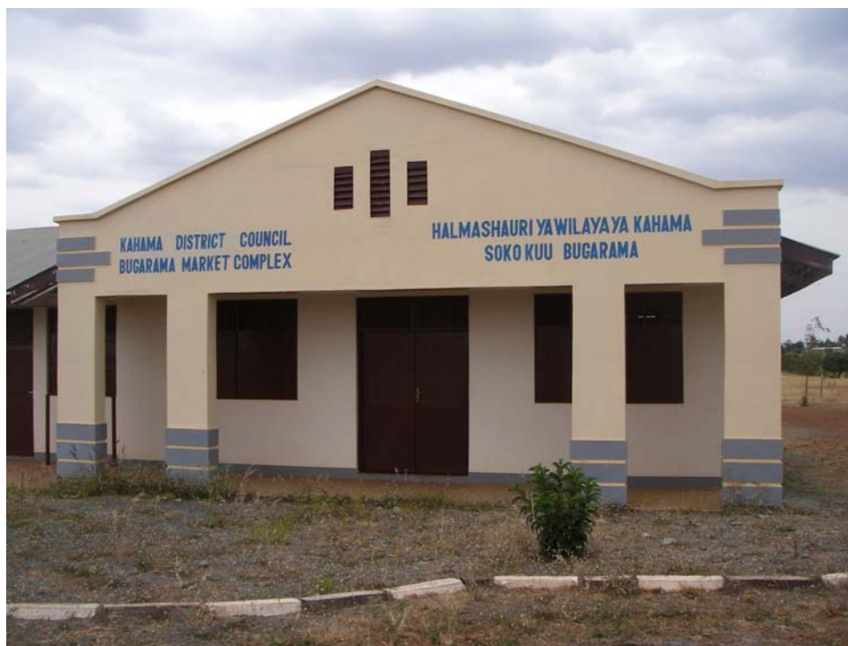
Fig. 5. 3 Newly constructed market complex at Bugarama.
