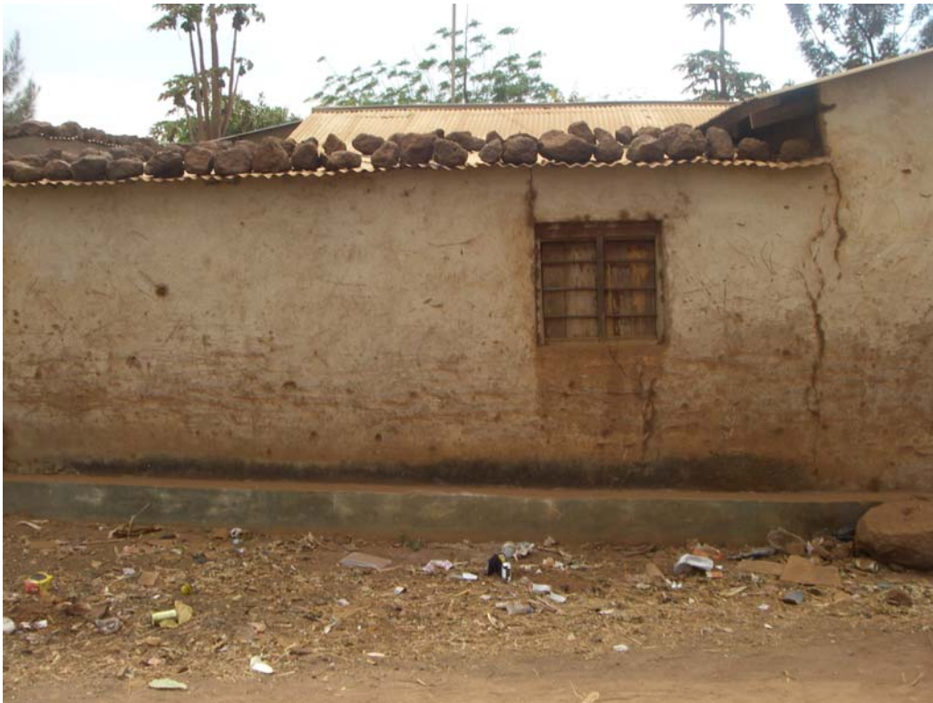
Fig. 5. 1 Most houses at Kakola centre have their roofs kept in place by stones
