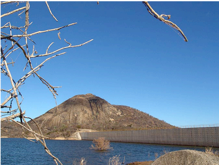
(Figure 9: Dam in the municipality of Bom Jesus da Lapa on the medium São Francisco river. Source: National Integration Ministry
