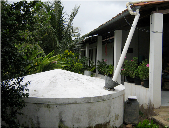
Figure 17: A rural cistern of the P1MC in the Northeast region. Source: ASA
