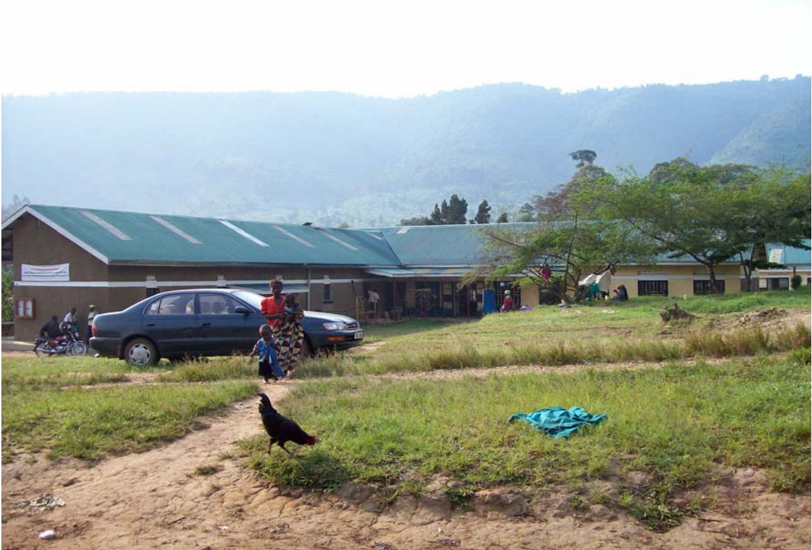
Plate 4 The administrative block and the main ward of BCHC Source: Field(Byaruhanga Michael)
