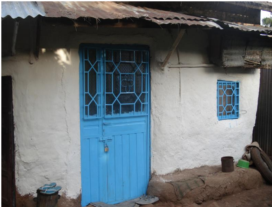
Figure 8: A typical returnee's house (Source: Author, fieldwork)
