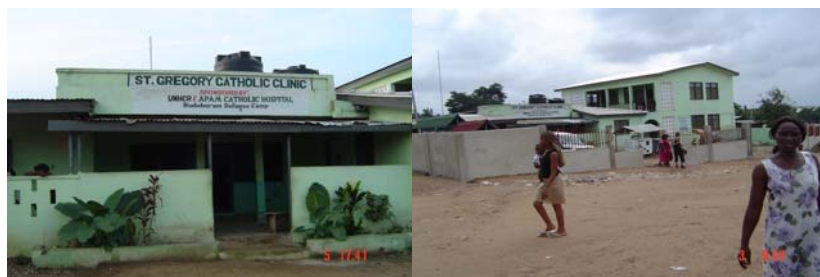
Fig. 7 Older Section of the Clinic on the Camp; Fig. 8 UNHCR-remodeled 2-storeyed extension of clinic
