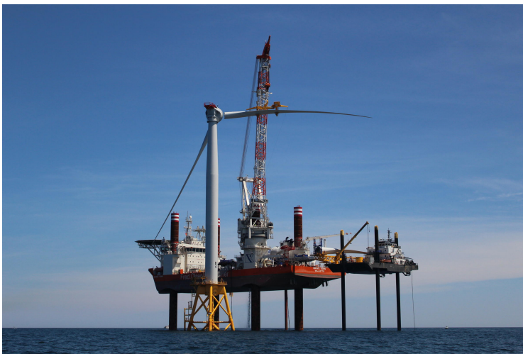
Figure 1. Single blade installation (Image source: RIPR [38]).
