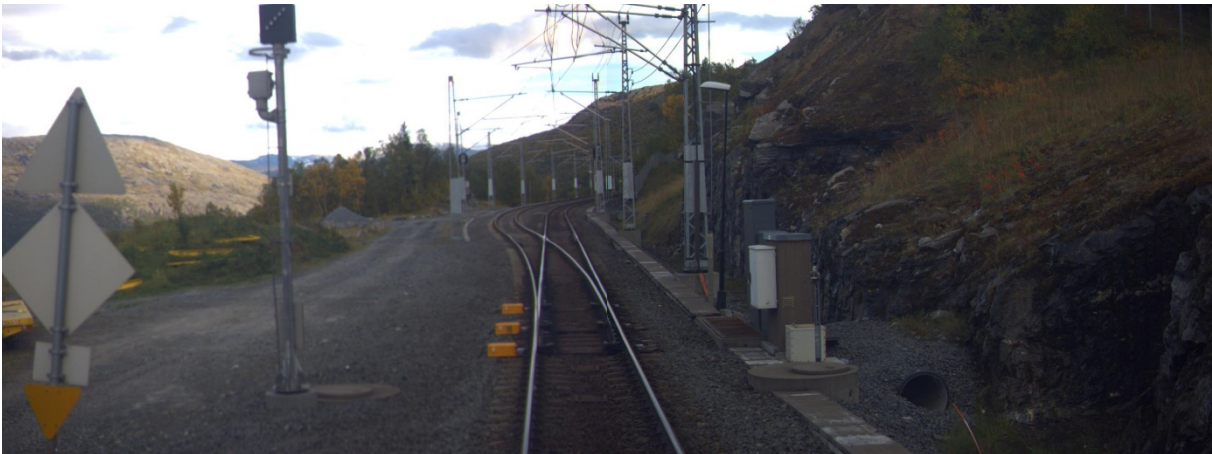
Figure 4-12 Ofoibanen km 13,04 (Bane NOR, 2017)
