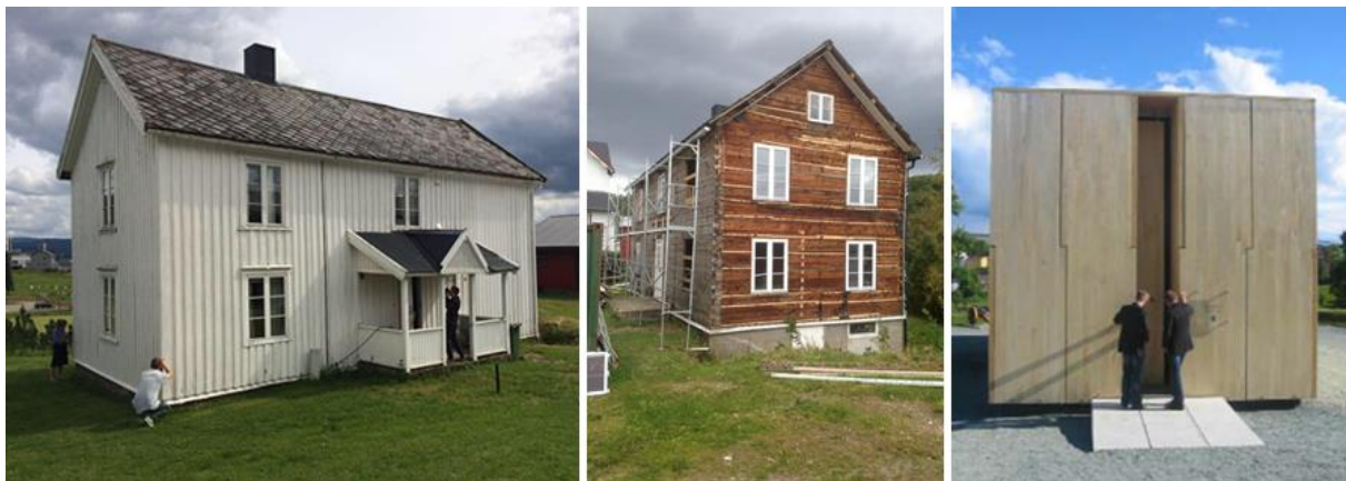
Figure 1 The log building from 1920s in original state (left), log building without external cladding (center), the artists pavilion in CLT from 2007 (right).
