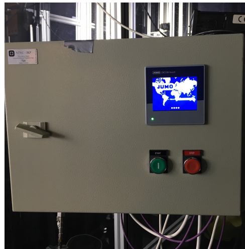
(c) The pump is switched on and off by pressing the green and red button respectively.
