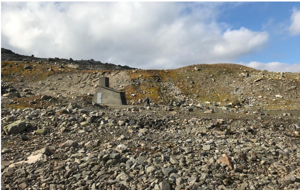
Figure 27. Gate house and the area covering the sink hole on the left backside of the gate house, seen as a terrain scar. Photo taken towards WSW, looking downstream the shaft, oblique to the weakness zone 17.
