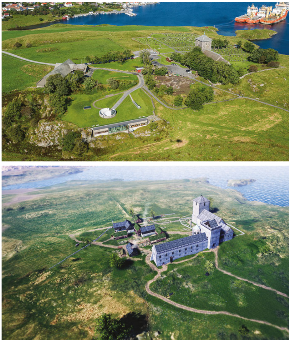
Fig. 8.2: Upper picture: Avaldsnes today with St Óláfr Church. Lower picture: reconstruction of how the royal complex at Avaldsnes might have looked around AD 1300. Photo: KIB Media. Reconstruction: R. Børshem/Arkikon.
