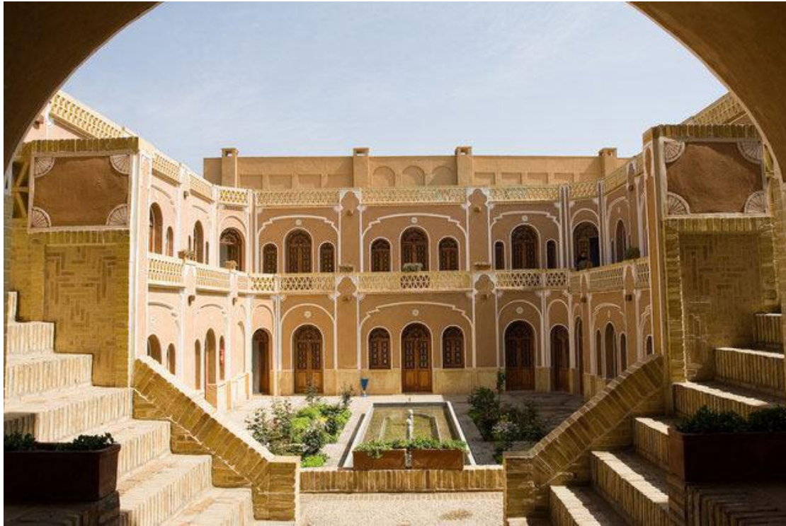
Fig. 1. A traditional building designed to receive the highest amount of solar energy in Yazd in winter.
