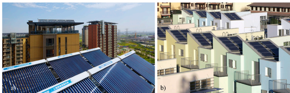
Fig. 15. a) Residential Plot B45 (CN) – Top view of the ST collectors on the roofs of the high-rise buildings' blocks (Source: © www.zhulong.com ). b) Violino District (IT) – Aerial view of the BIPV system on the roof of the 112 terraced houses (Source: © BAMSphoto - Basilio).
