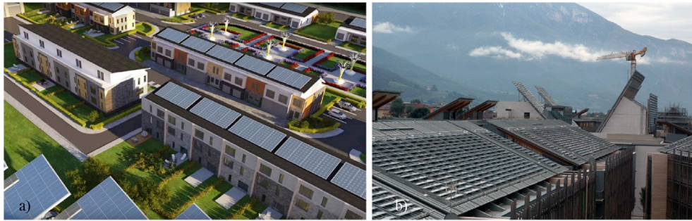
Fig. 19. a) London Solar Community Ontario (CA) - View of the PV panels installed on the roofs of the buildings (Source: © west 5). b) Le Albere (IT) - View of the polycrystalline PV modules integrated on the roof of the museum (Source: © S. Croce).
