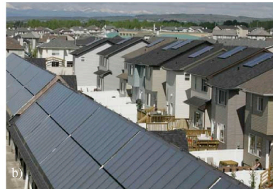
Fig. 18. Drake Landing Solar Community (CA) - a) Storage and solar heating system (Source: © www.dlsc.ca); b) View of ST collectors installed on the roofs. (Source: © CanmetENERGY, Natural Resources Canada).
