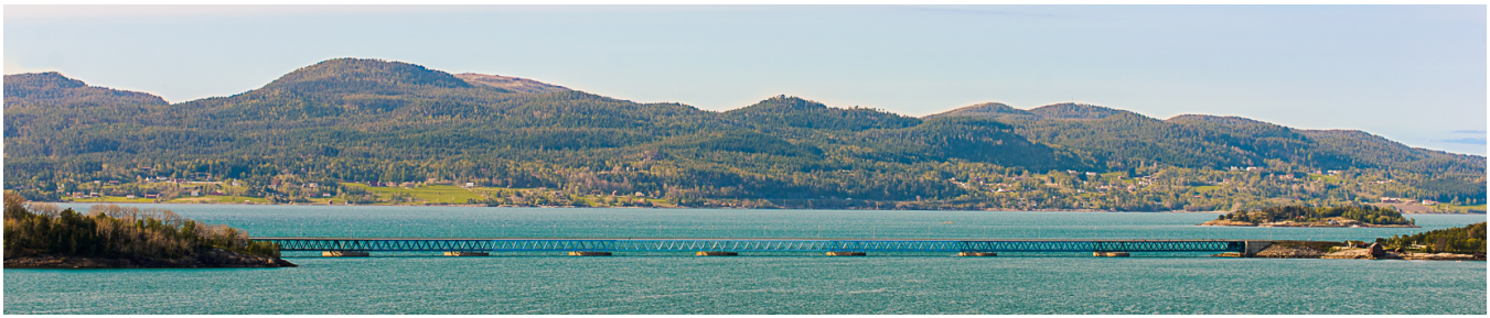
Figure 1: The Bergsøysund Bridge. Photograph by NTNU/K.A. Kvåle.
